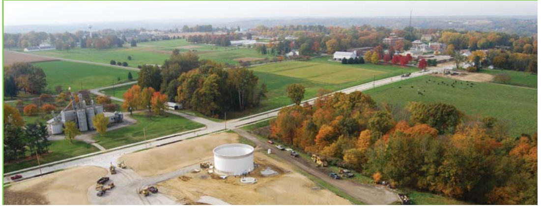
quasar's F550 system under construction on the OARDC campus
